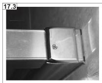
Silicone seal around OUTER edges of door and at junction of lower sill to wall frames on outer face. **Allow 24 hours before using shower.**
