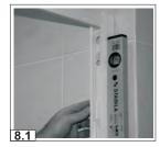
Re-fit clip-in extrusions, which were removed in stage 5.The Clip-in extrusion with "flipper seal" should be on the handle side of door. Ensure the leading edge is properly located along full height before pressing the Clip-in extrusion into the door frame, it will not locate properly if twisted. *Fig.* 9
