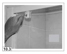
Adjust the door glass left or right so that it meets the closing seal evenly top to bottom and there is sufficient pressure on the edge of the glass to hold the door closed.
