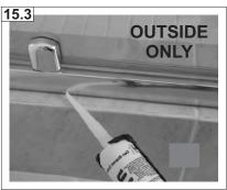
**Do not silicone seal on the inside of unit** (except where shown). Sealing the wallposts & sills to the tray on the inside can result in leakage problems- please note that, in use, water can penetrate into the frame extrusions- *this has no detrimental effect to the product*- however, this water must be allowed to drain out of the extrusions to the inside.
