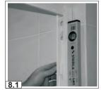
Re-fit clip-in extrusions, which were removed in stage 4. The clip-in extrusion with "flipper seal" should be on the handle side of door. Ensure the leading edge is properly located along full height before pressing the clip-in extrusion into the door frame, it will not locate properly if twisted. *Fig.* 9
